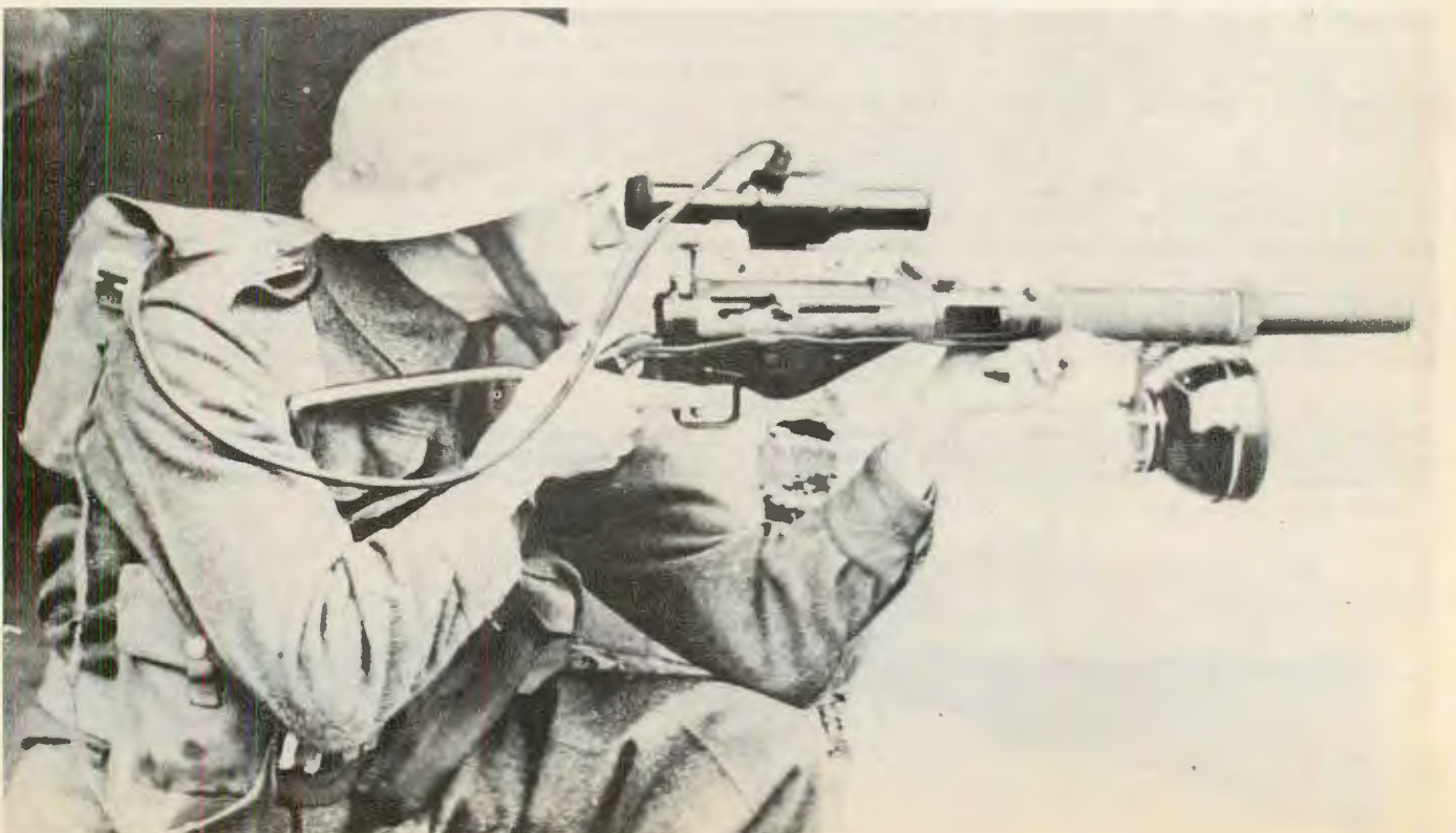
Below: An experimental special operations weapon, highly classified in its day. This sound-suppressed STEN was fitted with an infrared-light unit, and a telescopically-assisted infrared receiving unit. Device shown during field tests north of London, circa 1942. Photo courtesy the Imperial War Museum.
